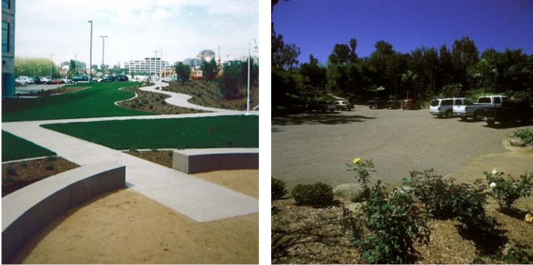
FIGURE 20. GRASSPAVE 2 FIRE LANE AND GRAVELPAVE 2 PARKING LOT (INVISIBLE STRUCTURES, INC.).
