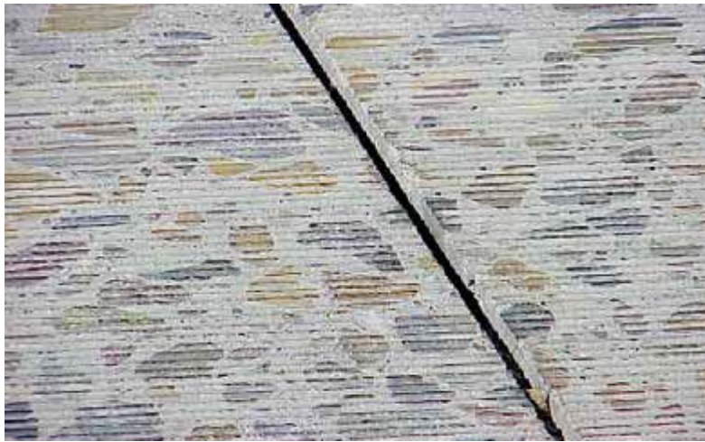
FIGURE 16. DIAMOND GRINDING (FELDMAN, 2009).
